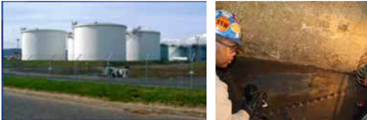
Figure 13. A technician in the field inspecting petrochemical storage tanks.
