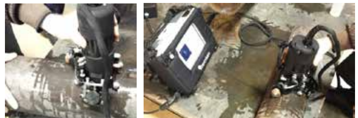
Figures 10 and 11. Inspection of a 6" steel pipe.
