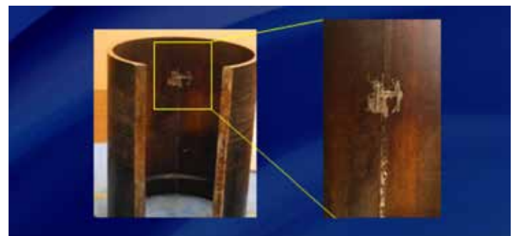
Figure 5: Steel pipe with “H” carved into rear side.
